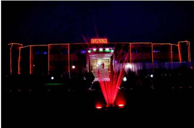
A view of DWSR administrative building
